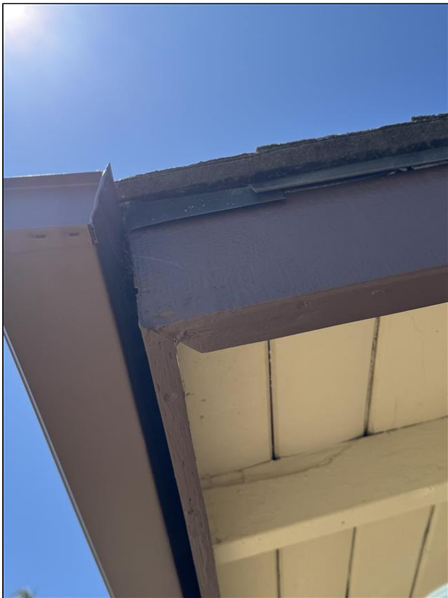
1.0 Item 5 (Picture) Eaves, Soffits, Trim 5
