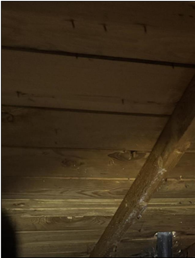
5.2 Item 1 (Picture) Sheathing 1
