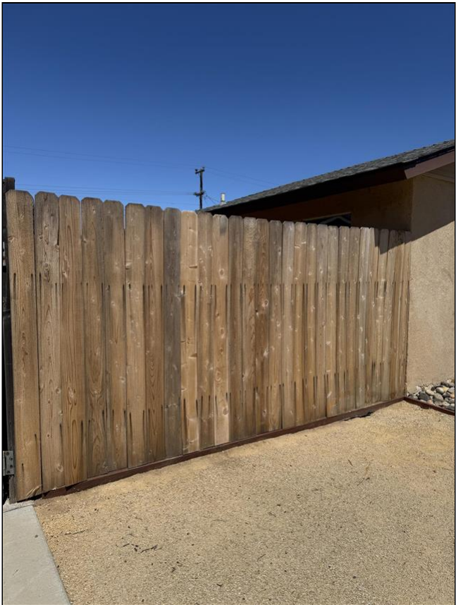
2.7 Item 2 (Picture) Left Front Fence
