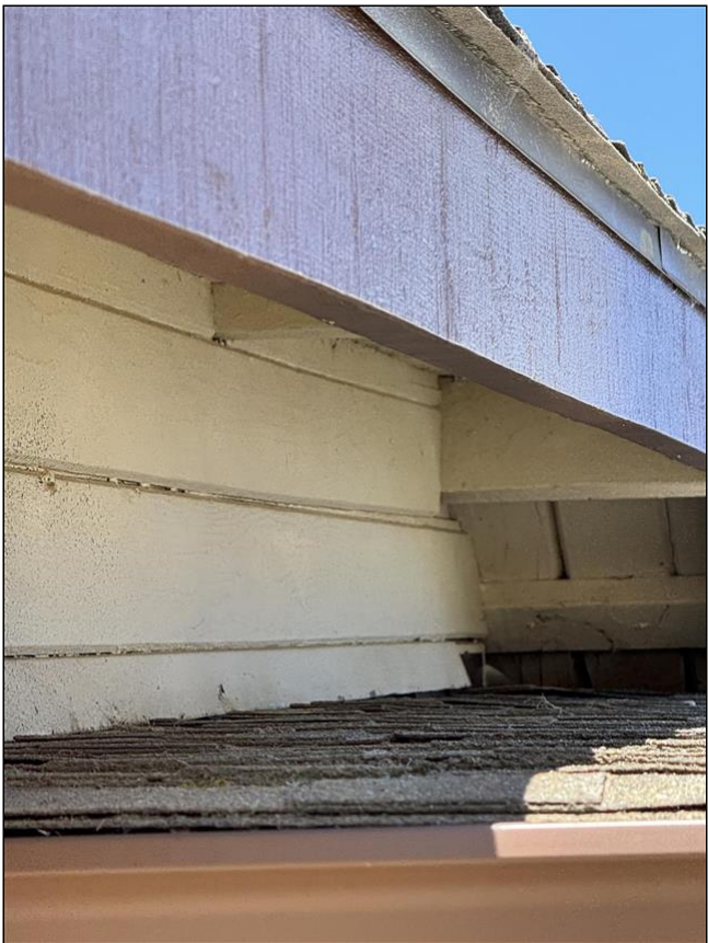
1.0 Item 6 (Picture) Eaves, Soffits, Trim 7
