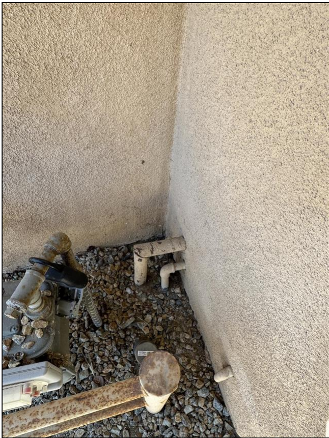
3.3 Item 3 (Picture) Stucco Walls
