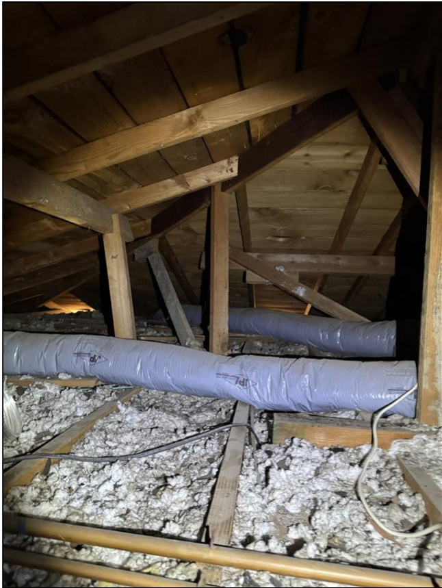
5.1 Item 1 (Picture) Conventional Framing 1
