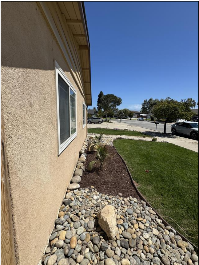
2.0 Item 2 (Picture) View 3
