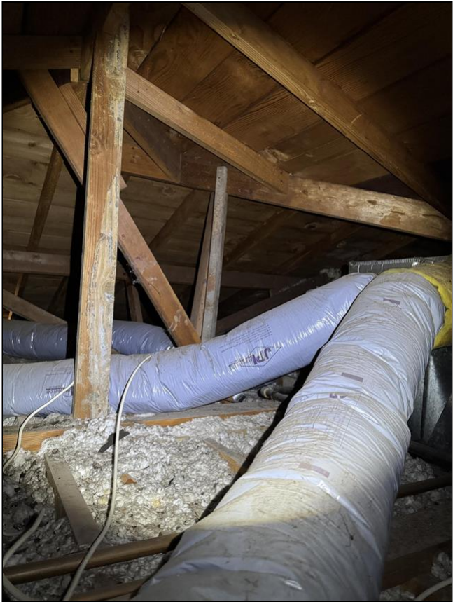
5.1 Item 2 (Picture) Conventional Framing 2
