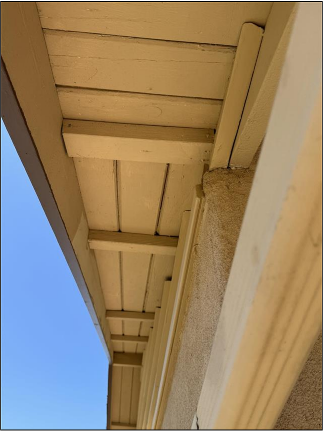
1.0 Item 8 (Picture) Eaves, Soffits, Trim 9
