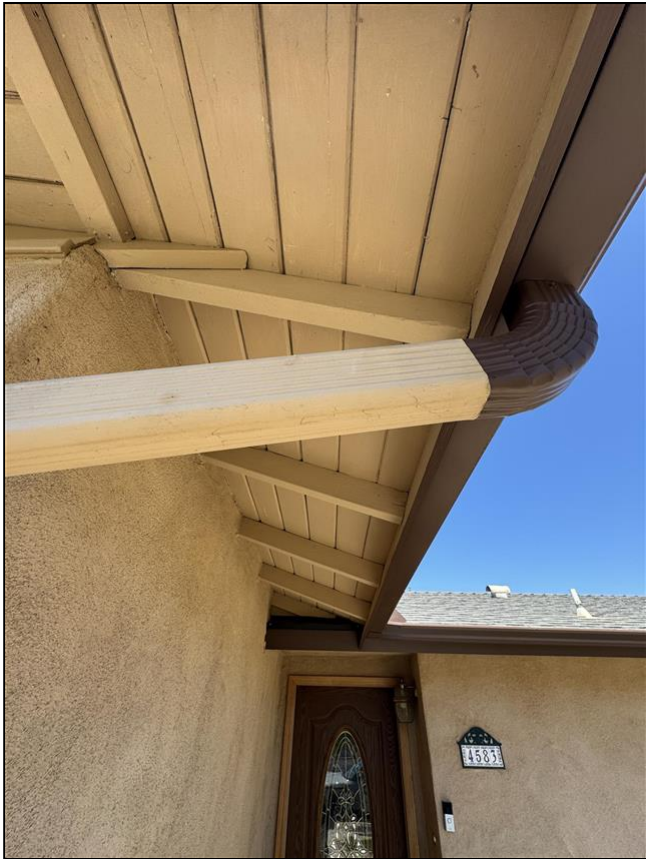
1.2 Item 1 (Picture) Downspout and Gutter
