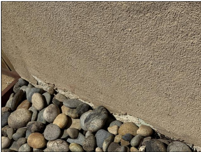
4.0 Item 1 (Picture) Bottom of Front Wall
