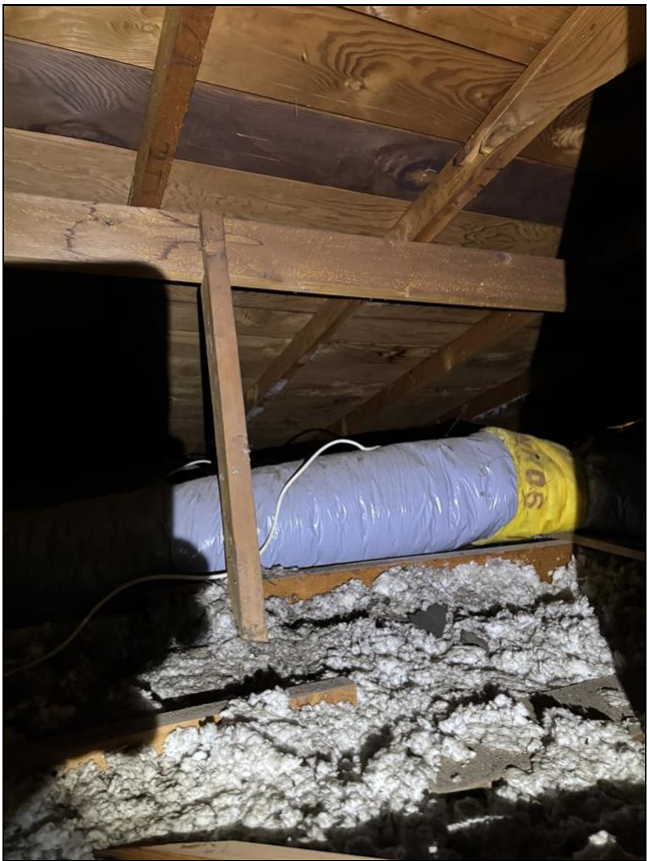
5.1 Item 4 (Picture) Conventional Framing 4
