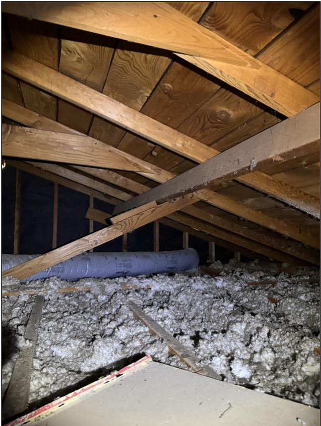
5.0 Item 2 (Picture) Attic 1
