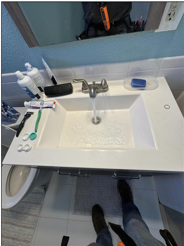
11.8 Item 1 (Picture) Sink 1
