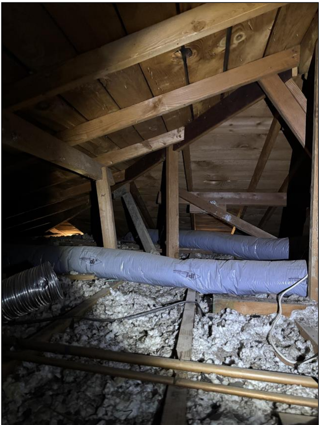
5.1 Item 6 (Picture) Conventional Framing 6
