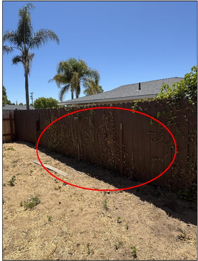
2.7 Item 6 (Picture) Rear Fences with Vine Material
