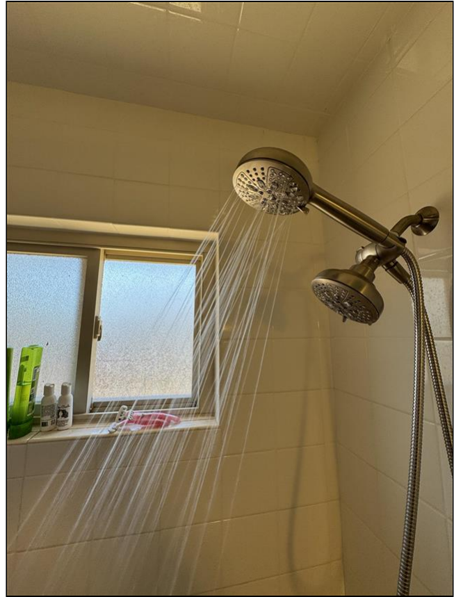
11.7 Item 2 (Picture) Hallway Shower
