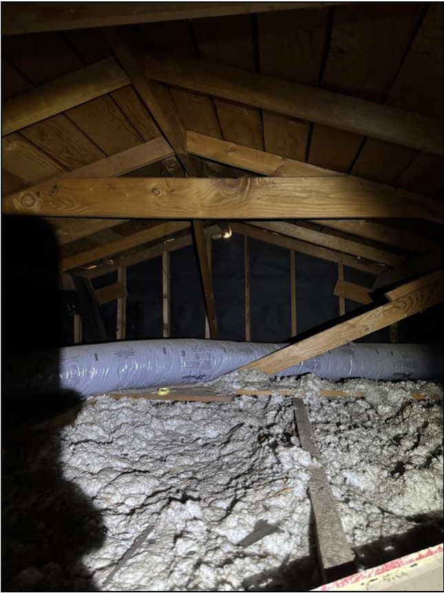
5.0 Item 3 (Picture) Attic 2
