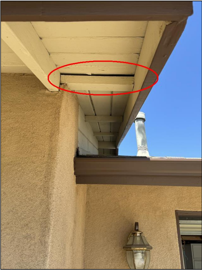
1.0 Item 7 (Picture) Eaves, Soffits, Trim 8
