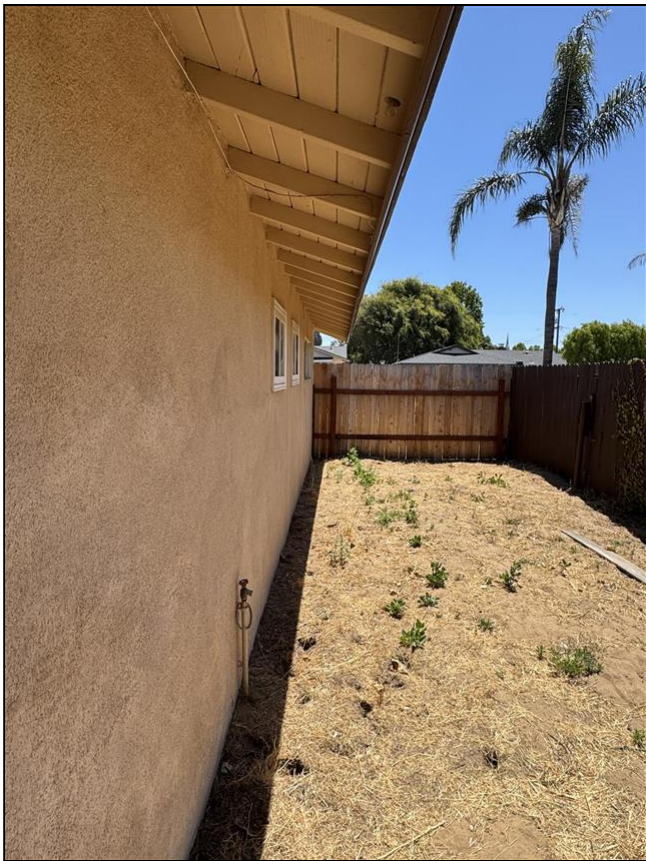
2.0 Item 3 (Picture) View 4
