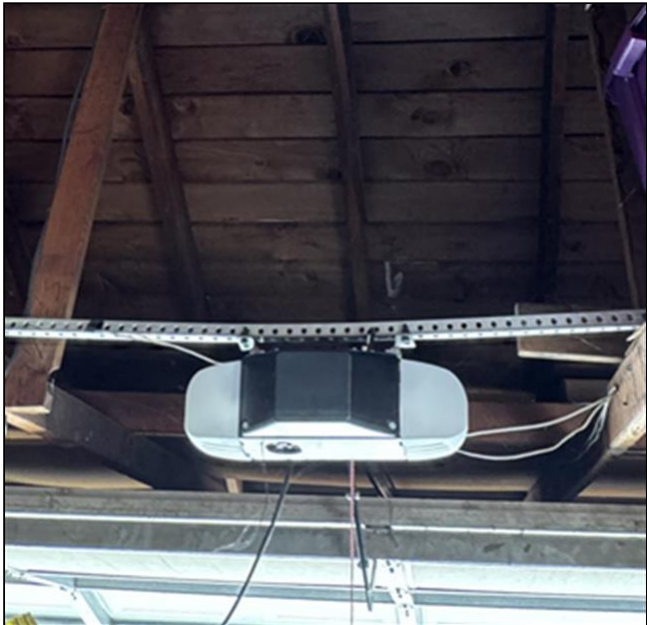
7.0 Item 1 (Picture) Door Opening Garage
