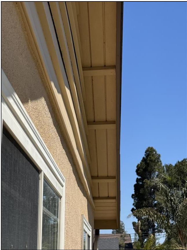
1.0 Item 3 (Picture) Eaves, Soffits, Trim 3
