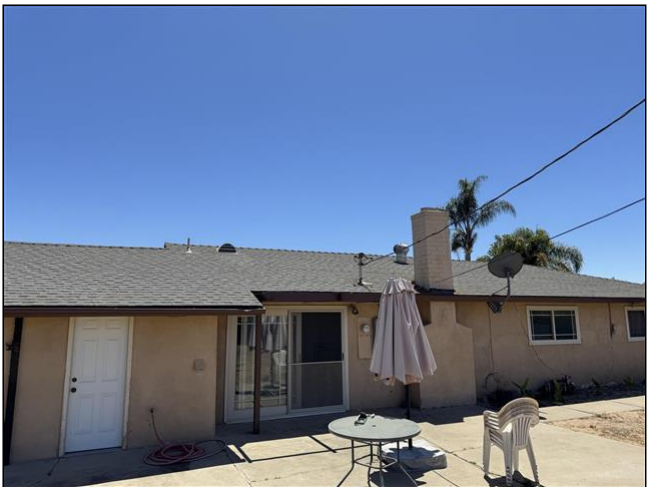
2.0 Item 6 (Picture) View 7
