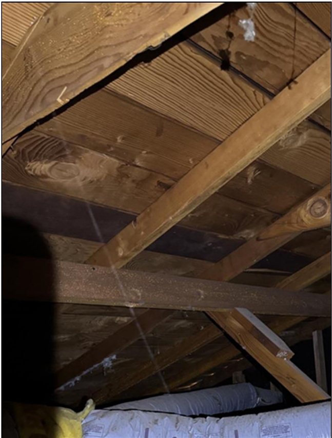
5.2 Item 2 (Picture) Sheathing 2
