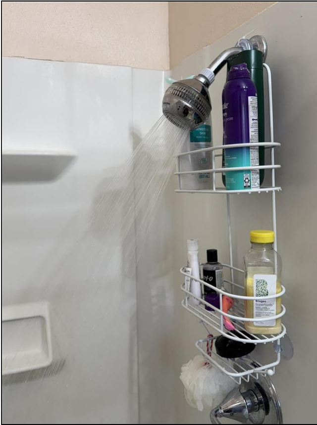
11.7 Item 1 (Picture) Master Shower
