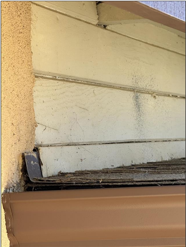
1.1 Item 2 (Picture) Flashing 2
