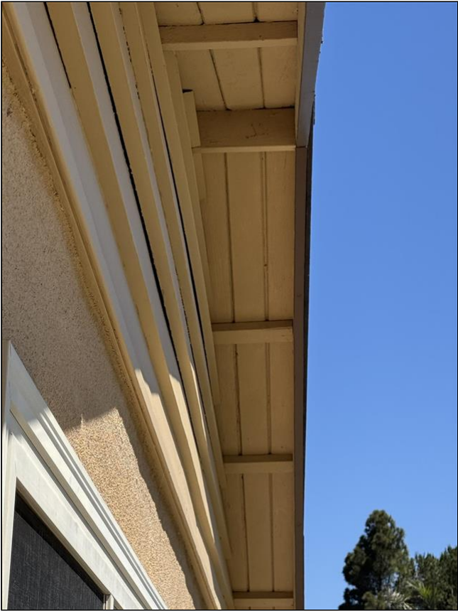
1.0 Item 9 (Picture) Eaves, Soffits, Trim 10
