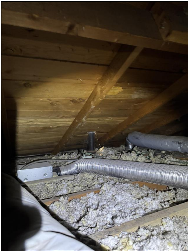
5.1 Item 3 (Picture) Conventional Framing 3
