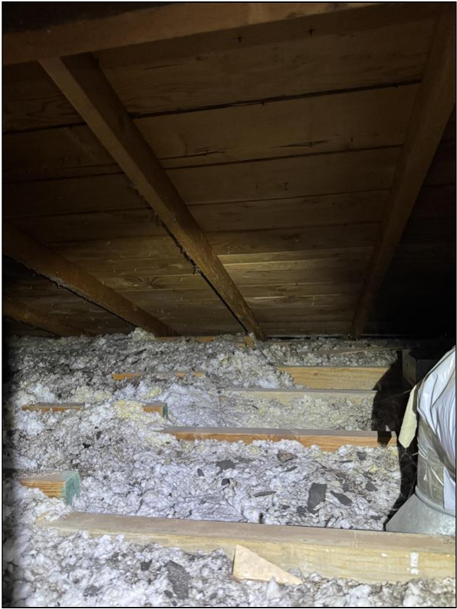
5.0 Item 4 (Picture) Attic 3
