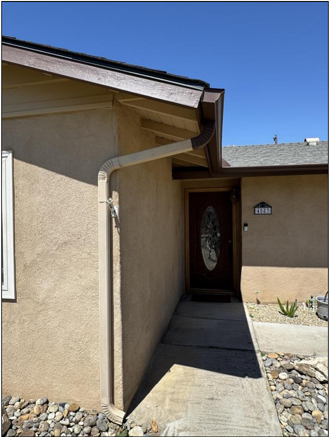
1.2 Item 2 (Picture) Downspout
