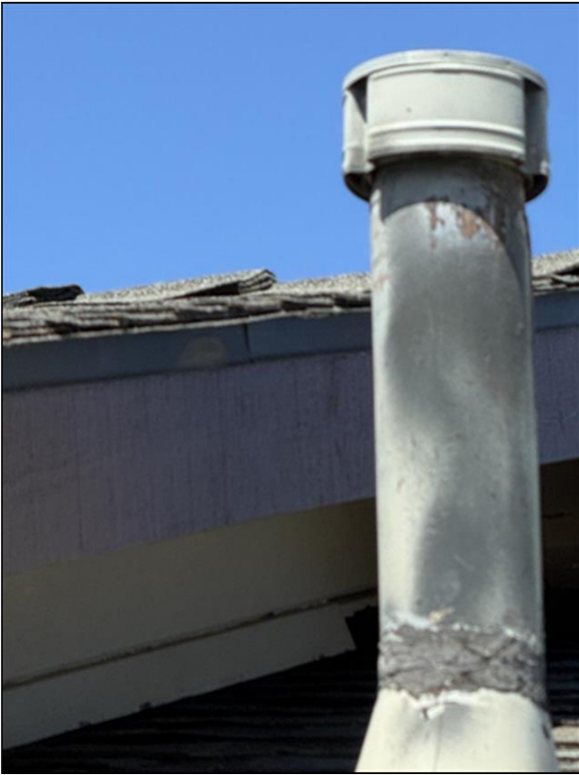
1.1 Item 3 (Picture) Flashing 3
