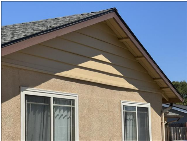
1.0 Item 1 (Picture) Eaves, Soffits, Trim 1
