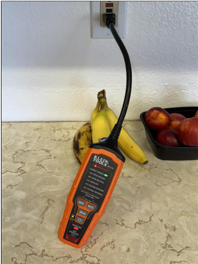
6.5 Item 1 (Picture) GFCI 1
