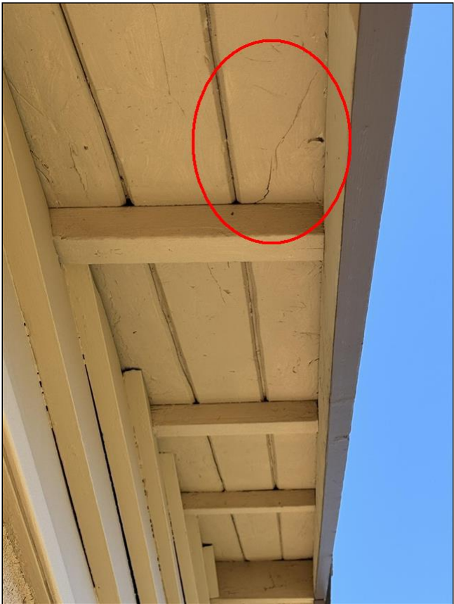
1.0 Item 2 (Picture) Eaves, Soffits, Trim 2
