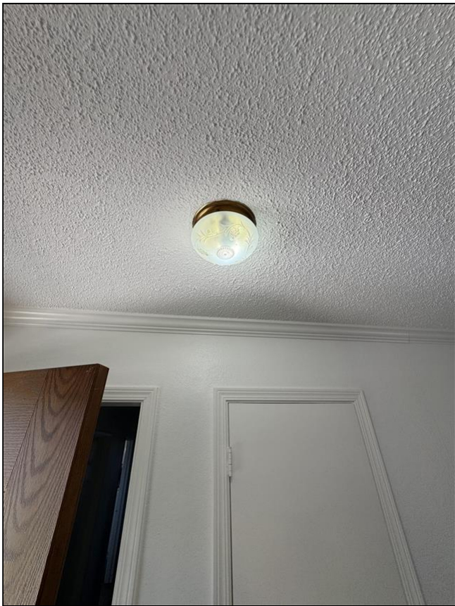
6.7 Item 7 (Picture) Bedrooms Light 2
