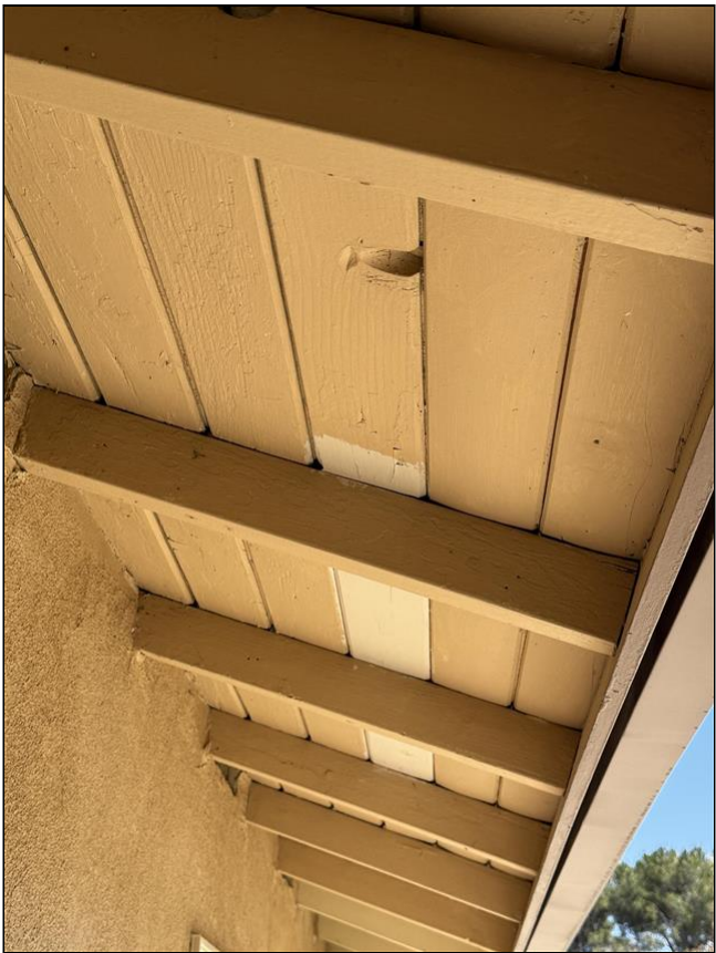
1.0 Item 4 (Picture) Eaves, Soffits, Trim 4
