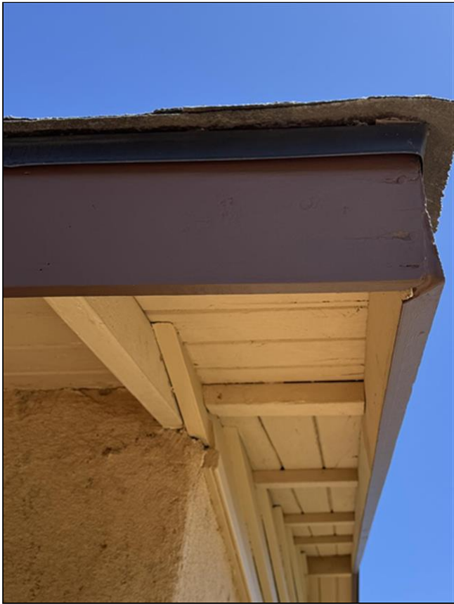
1.1 Item 1 (Picture) Flashing 1
