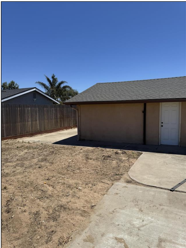
2.0 Item 5 (Picture) View 6
