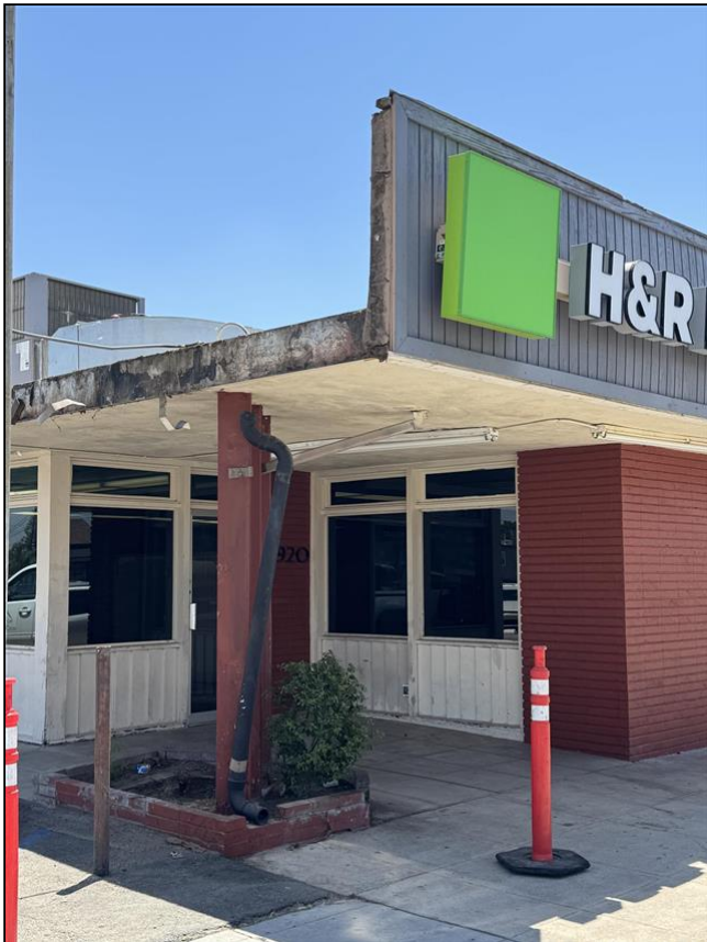
1.0 Item 1 (Picture) Front Corner
