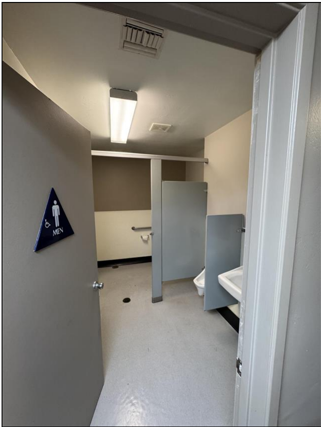
8.1 Item 3 (Picture) Bathroom Ceiling
