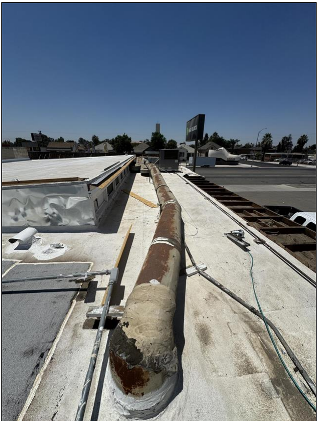
2.0 Item 2 (Picture) Front Roof
