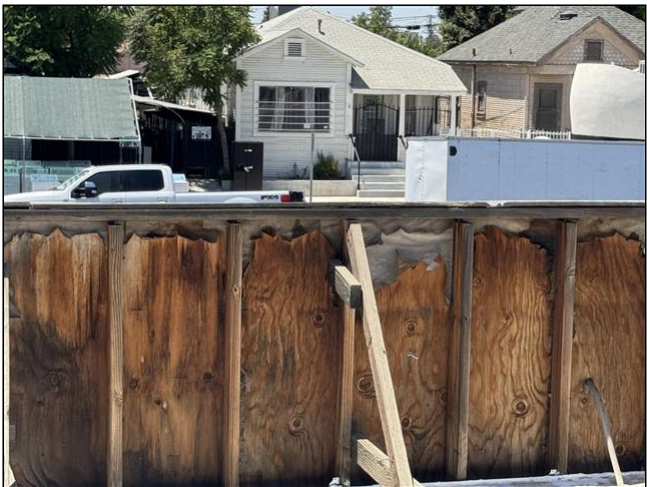
2.0 Item 6 (Picture) Street Facing Facade
