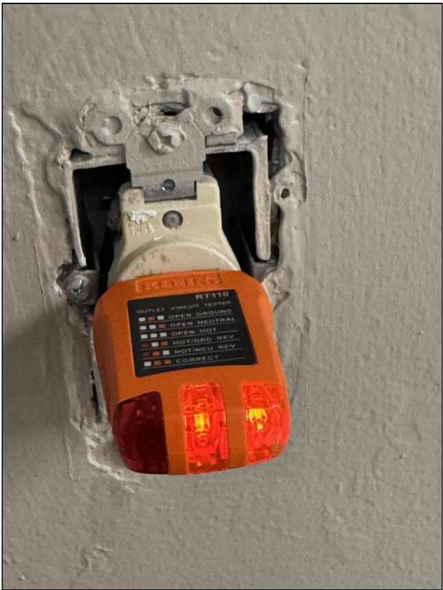
6.0 Item 8 (Picture) Media Missing Plate
