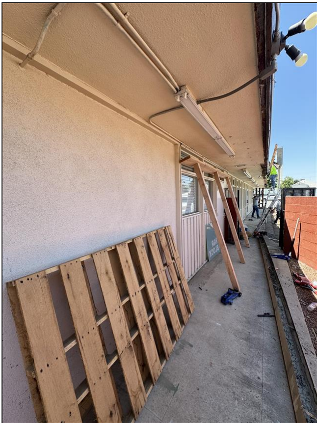
3.5 Item 3 (Picture) Walkway 3
