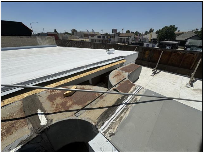
2.0 Item 8 (Picture) A/C Vents
