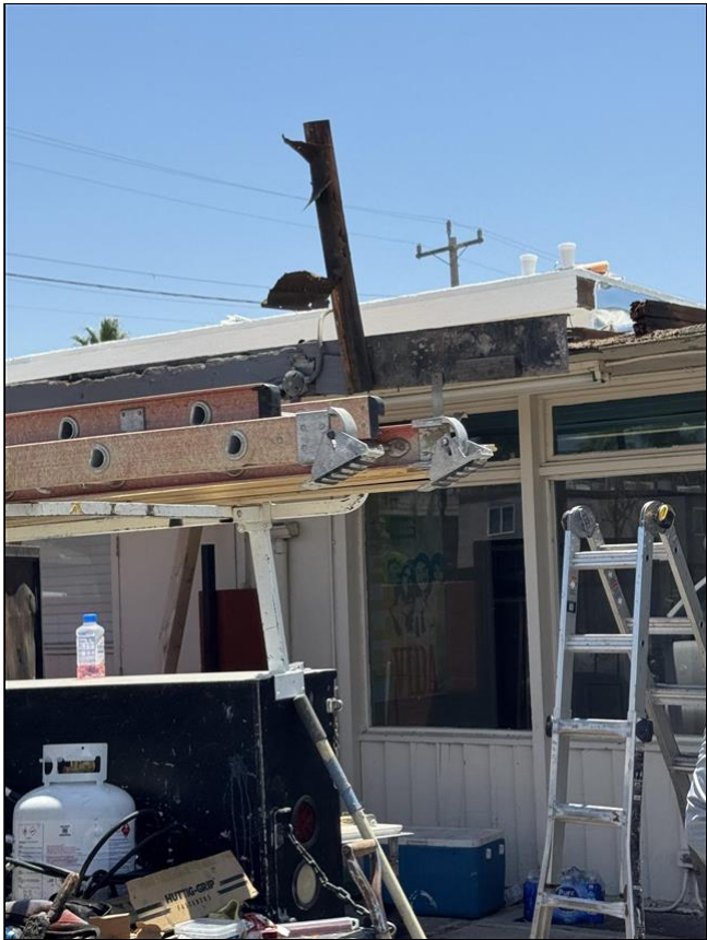
3.0 Item 1 (Picture) Roof and Overhang Work
