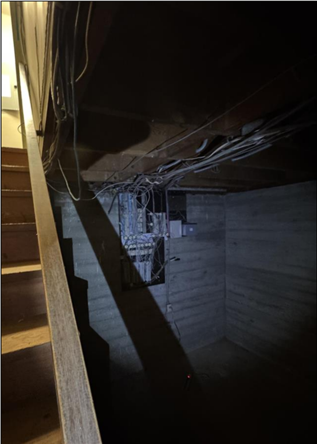
6.0 Item 13 (Picture) Old Comm Basement
