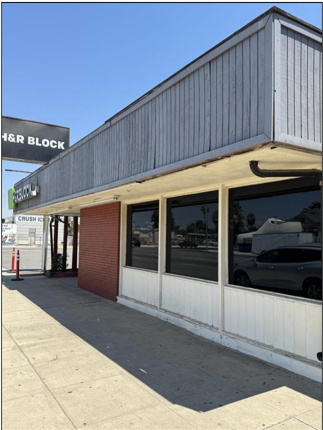
3.5 Item 2 (Picture) Walkway 2
