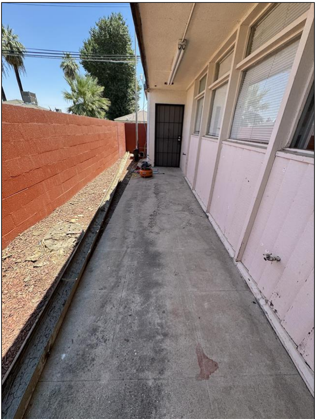
3.5 Item 4 (Picture) Walkway 4
