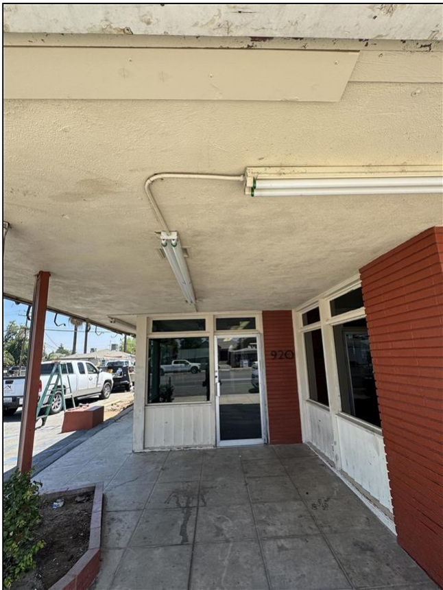
3.5 Item 1 (Picture) Walkway 1
