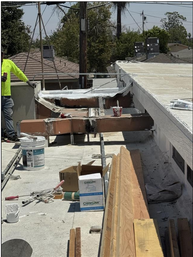
2.0 Item 5 (Picture) Roof Work
